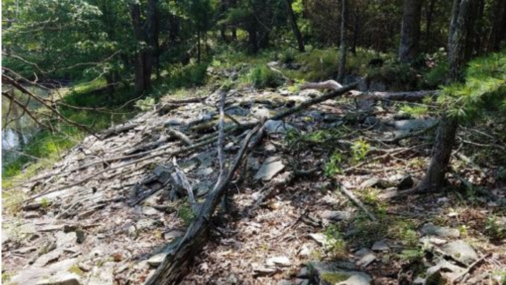
Photo 11. View looking west of embankment separating water bodies E and F.
